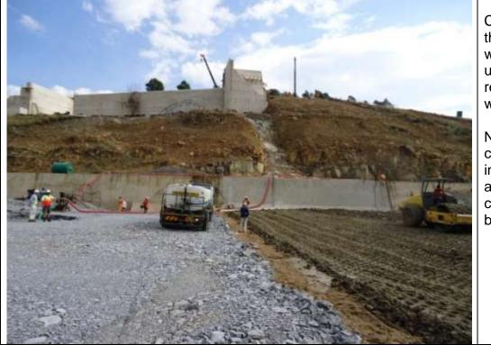
Construction of the rockfill dam with clay core underway, after repair of coffer wall.
