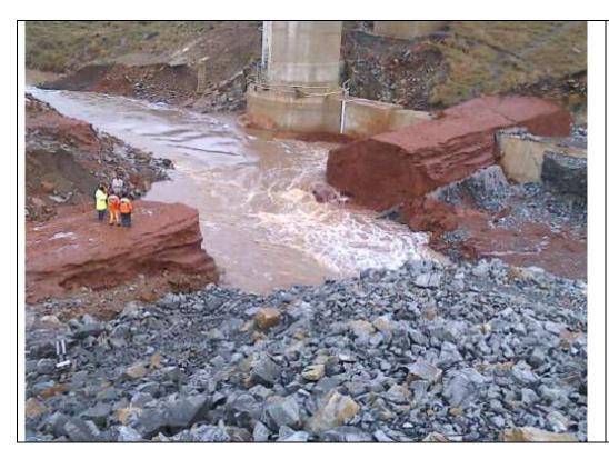
Failure of coffer wall after being overtopped by a small flood.
