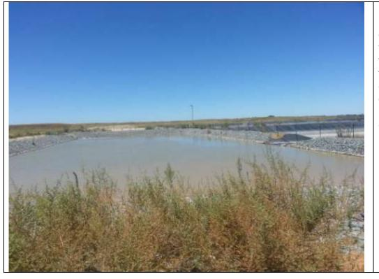
Return water dam. Filtered water is transported through pipes to existing tailings dams to make more sludge for gold processing. Modderfontein Factory Dams 1, 3, & 4 owned by Heartland Leasing Pty (Ltd). This is an example of feedback from the owner on progress made of implemented recommendations from the 5 yearly Dam Safety Inspection Report.
