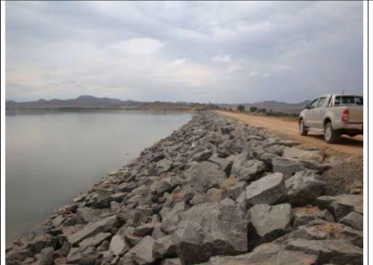
Rehabilitation of the upstream face showing the new rip rap already at crest level. A gravel layer at crest level is still outstanding.
