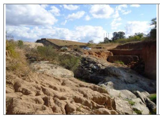
Erosion damage occurred in the spillway channel, encroaching towards the earthfill dam wall in the background.
