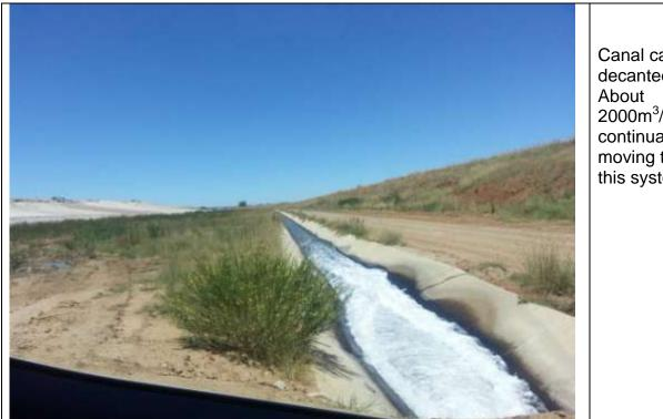
Canal carrying decanted water. 2000m<sup>3</sup>/hr is continually moving through this system.
