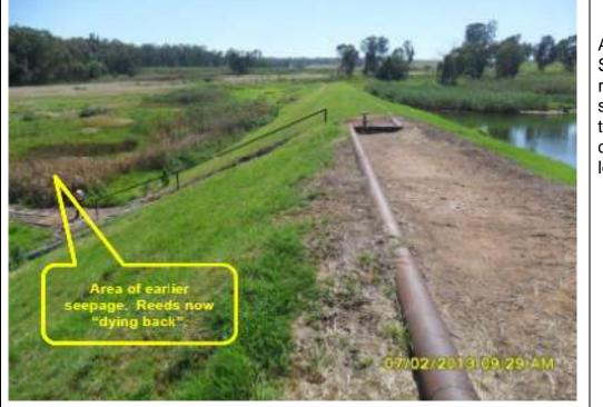
AFTER: Seepage has reduced substantially due to the lowering of the dam water level.
