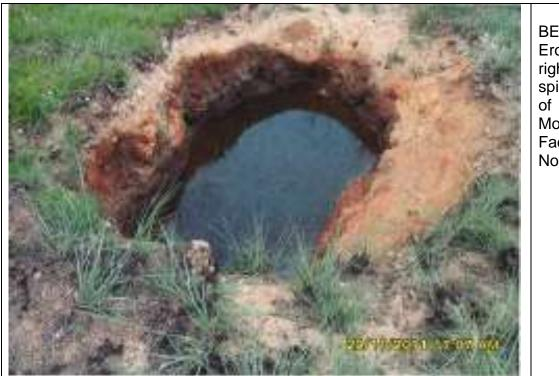
BEFORE: Erosion hole in right bank spillway chute of Modderfontein Factory Dam No 3.
