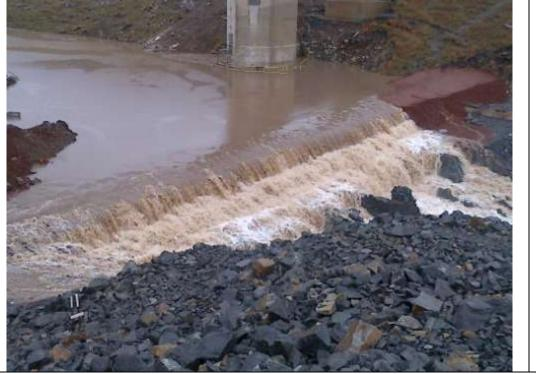
Coffer wall being overtopped by small flood, when discharge capacity of diversion pipe was exceeded.
