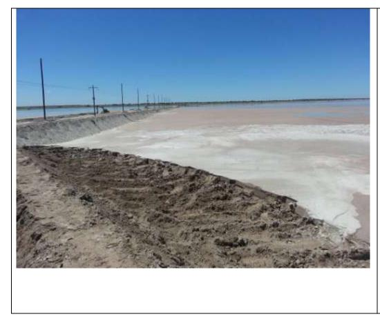
About 1000m<sup>3</sup>/hr of sludge is transported from exisiting/ decommissione d tailings dam to a pumpstation onto the Chemwes Kareerand Tailings Mega Dam and deposited via cyclones.
