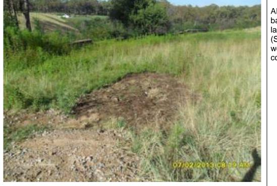
AFTER: Hole backfilled in layers. (Soilcrete and well compacted)
