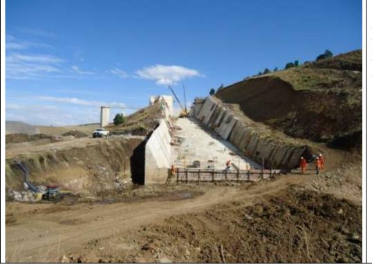
Picture of downstream part of side-channel spillway. Soil nails were used to anchor side walls.
